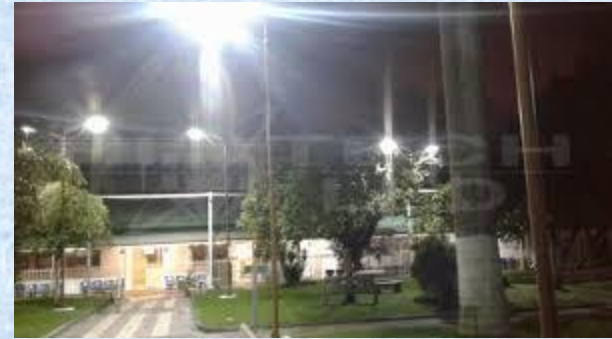
Private road lighting
